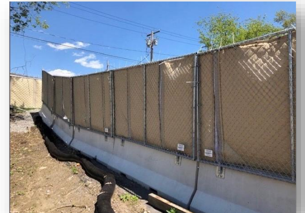
Fenced Work Area
